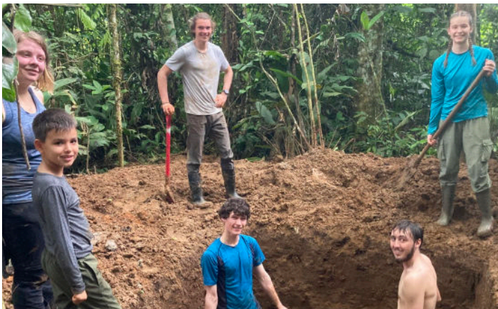
Outhouse hole digging!
